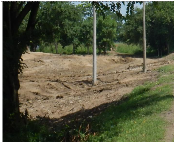
R2. VISTA GENERAL
