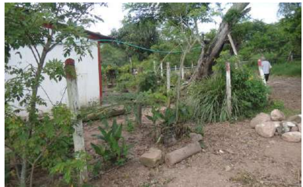
B4: Cerca perimetral
