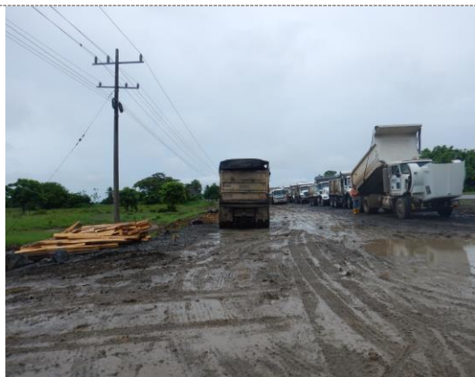
R1. VISTA GENERAL
