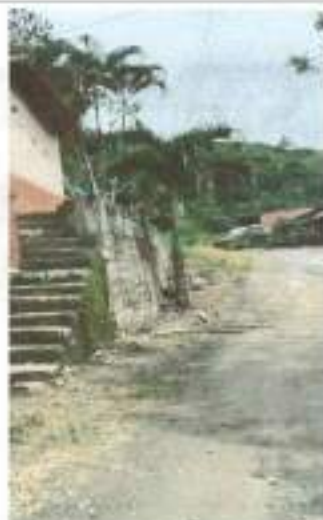
CA1: MURO PERIMETRAL
