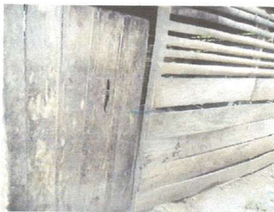
CA16: ENRAMADA 4 - FACHADA
