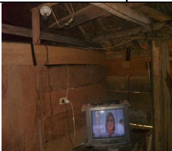
Vista interior C1
