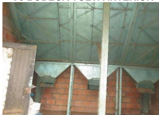
C6 BODEGA TOLVA INTERIOR
