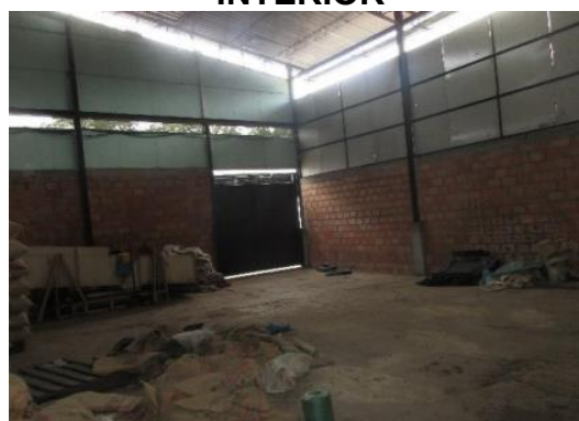
C4 BODEGA TRILLADORA INTERIOR
