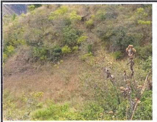
Vista general interna
